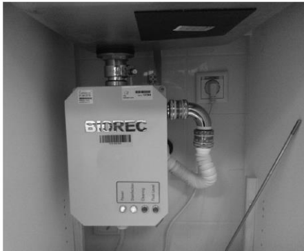
Figure 1. The self-disinfecting Medizinische Hygiene-Siphon BIO-REC (MoveoMed, Dresden, Germany).
